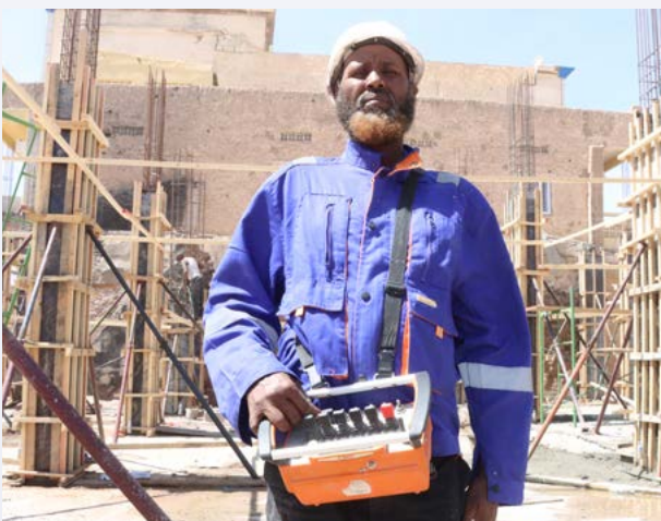
Pharo Construction employee rebuilding the Waheen Market that was hit with massive fire on April 1st, 2022. The market is located in Hargeisa, Somaliland.
