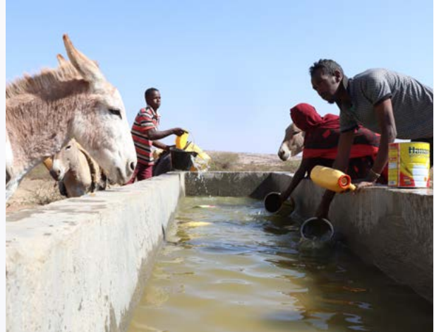
Community members using the rehabilitated Illinta Hafir Dam in Somaliland.
