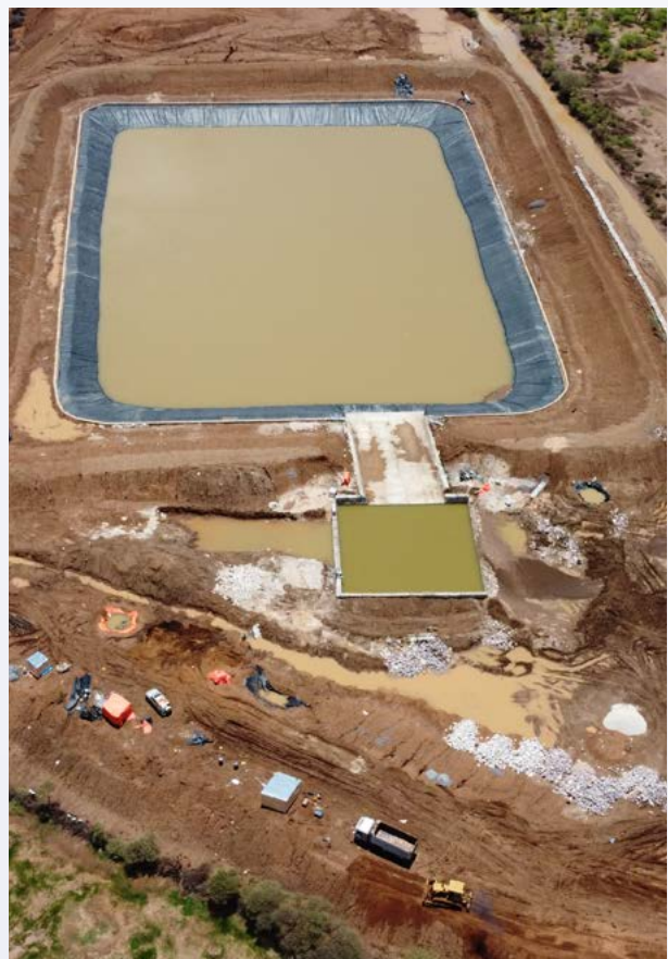
An ariel view of the Illinta Hafir Dam after the rains.
