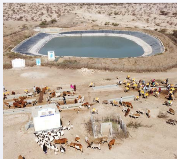
Aerial footage of Illinta dam (75.5mX57mX4m) located in Gabiley, Somaliland. With storage capacity of 17,400.00 cubic meters that will provide clean and adequate water for 247 households through the year particularly during the dry season.
