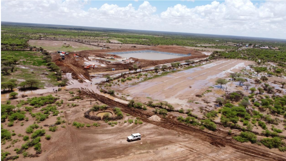
Wado-Makahiil dam under construction
