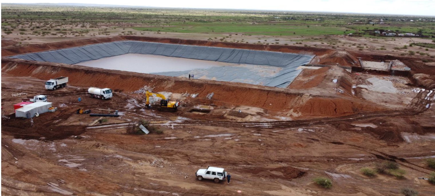
Ijaara dam under construction
