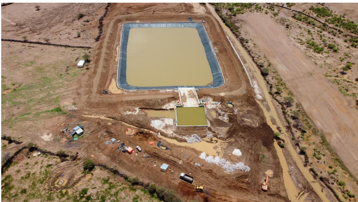
Wado-Makahiil dam filling with water
